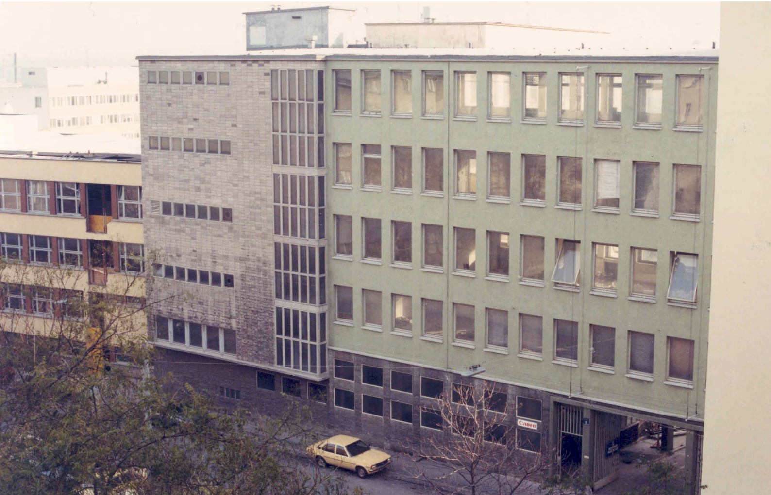
Before its adaptation for research, the future IMP site housed a 1950s factory building used by the Hornyphon electronics company.
